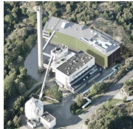
120 GJ SNG pilot plant
