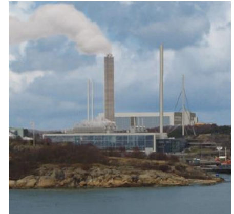
500 GJ SNG scale-up plant
