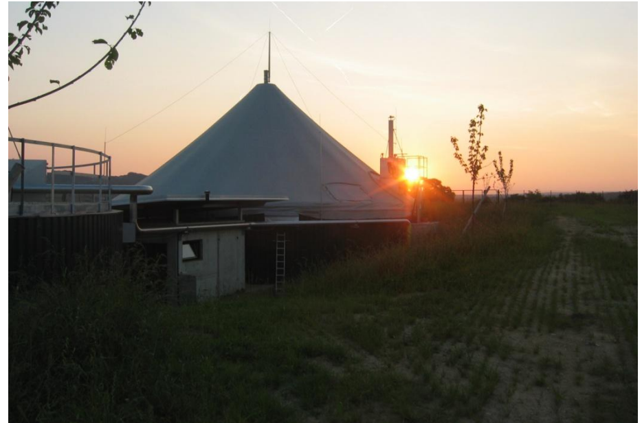
ph & temperature-controlled digester in Strem /Guessing District, at European Centre of Renewable Energy (Future Energy Technologies)
